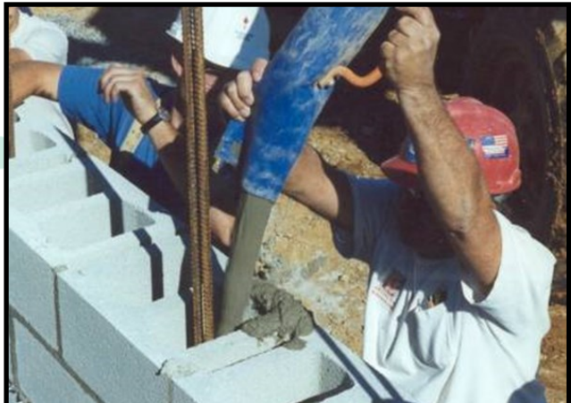
Placing Grout in Masonry Block
